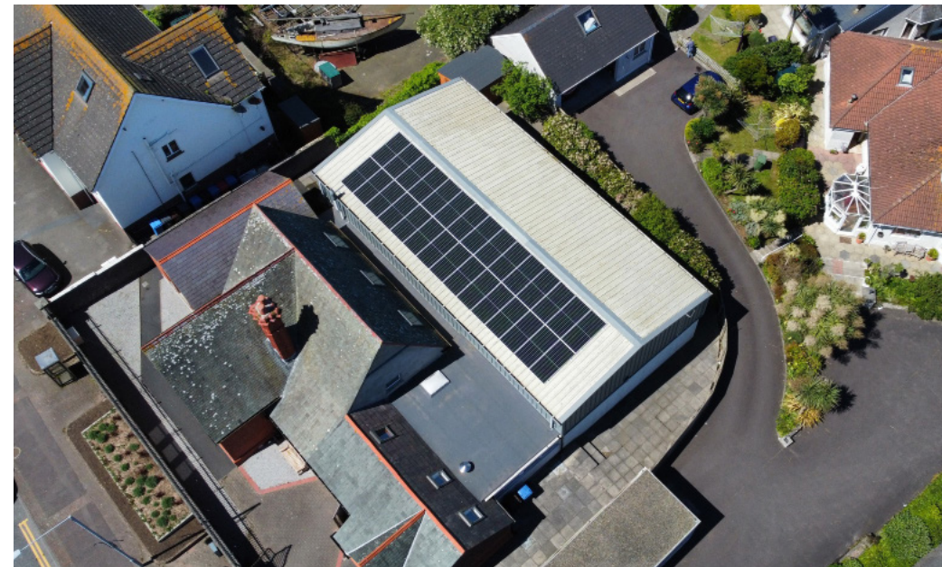
The solar panels on the Canon Tyney Hall
